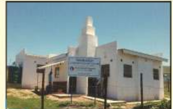
ISLAMIC CENTRES CONSTRUCTION
