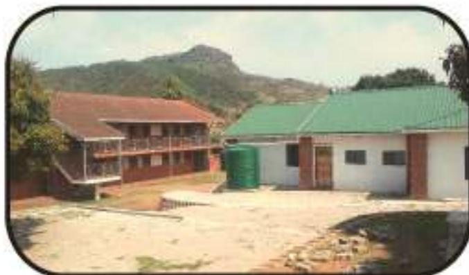
Zilweleni Islamic Centre Water Tank
